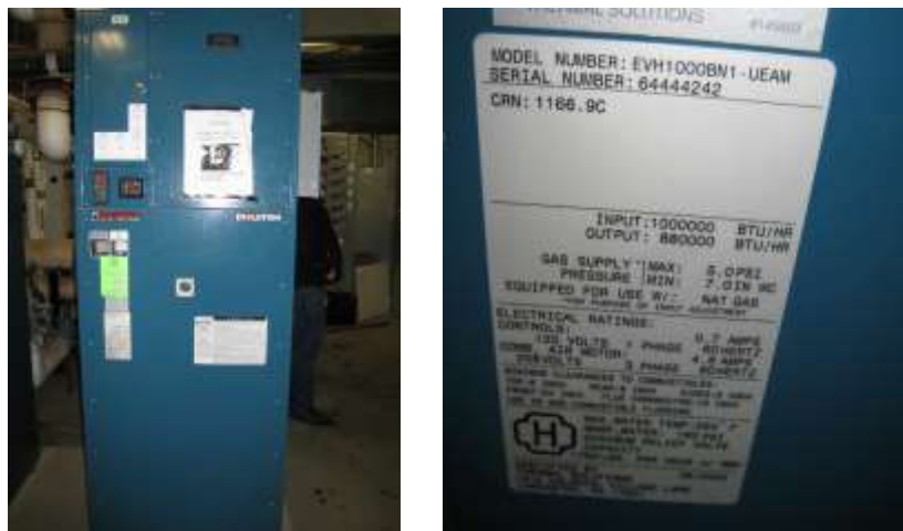
Figure 5: Thermal Solutions Boiler
